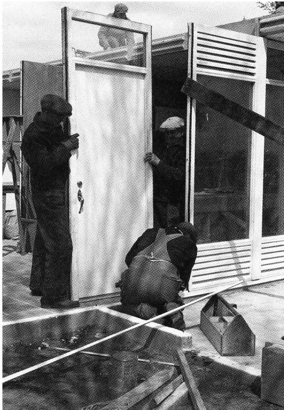
127, 128 Green's Ready-Built, construction in progress, 1946
