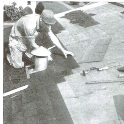
Roofing materials go down faster over solid PlyScord sheathing. Factory seasoning assures dimensional stability. PlyScord won't shrink or swell like boards to damage roofing. Roofing lays flat, stays flat. PlyScord roof sheathing adds strength and rigidity, acts as a structural diaphragm in resisting loads caused by high winds, earthquakes.
