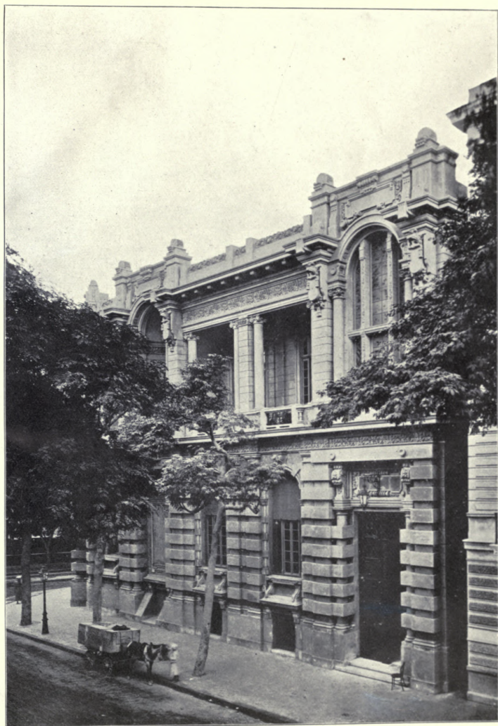
National Bank of Egypt, Cairo, FABRICIUS PASHA, Architect.
