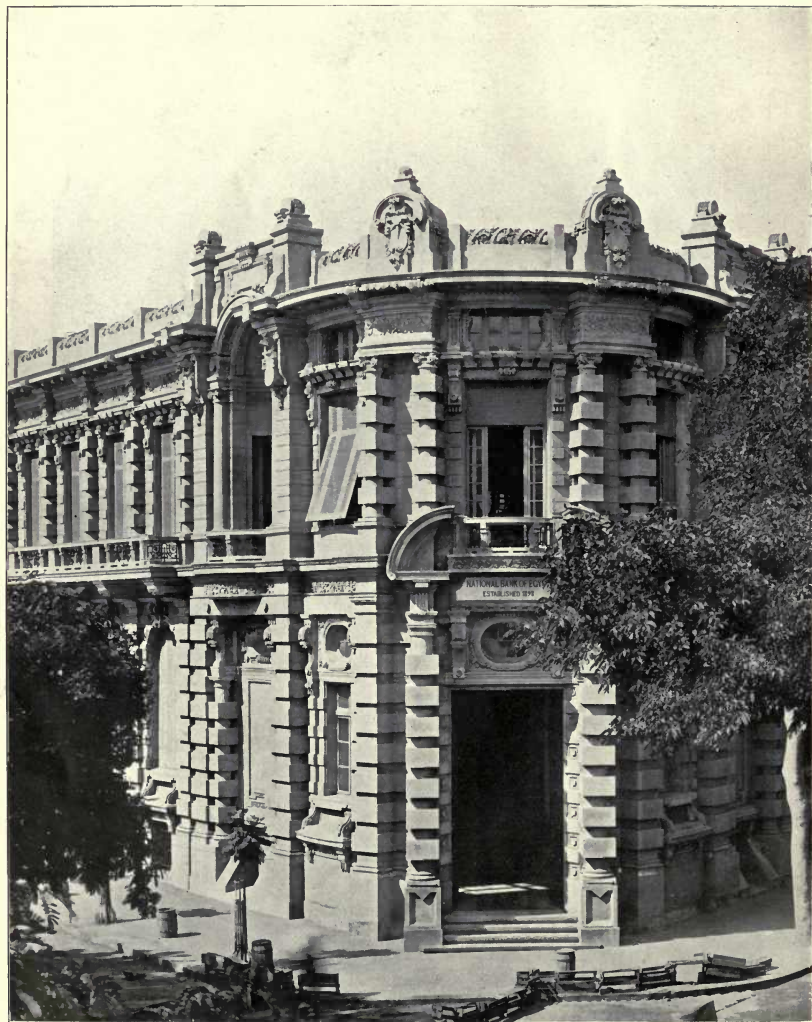
National Bank of Egypt, Cairo, FABRICIUS PASHA, Architect.
