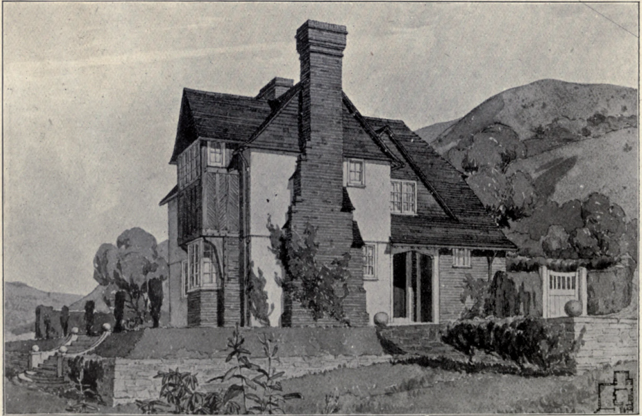
Cottage at the School of Lady Gardeners, Glynde, GEOFFREY LUCAS, Architect. (For Plans, see p. 121.)
