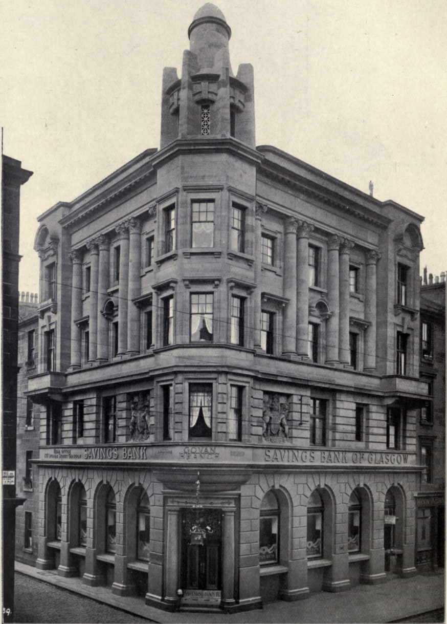
791. Savings Bank of Glasgow, Gowan Branch, ERIC A. SUTHERLAND, Architect. Mason: G. Barlas and Co., 13 Ruthven Street, Hillhead, Glasgow. Joinery: John Cochrane, 58-70 Dobbies Loan, Glasgow. Marble: Galbraith and Winton, 185 St. Vincent Street, Glasgow. Heating: Cameron and Co., Glasgow.
