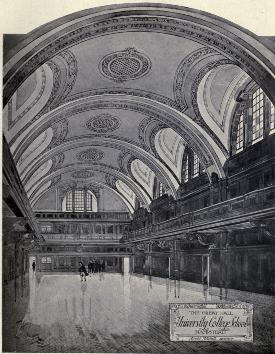
1609. University College School, Hampstead, Great Hall, ARNOLD MITCHELL, Architect. Builders: Dove Bros., 15 Studd Street, Islington, N.
