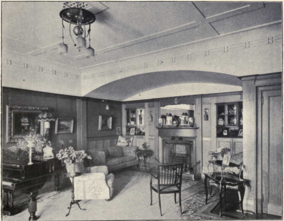
808. Terrace House, Montgomerie Drive, Kelvinside, Glasgow, J. C. McKELLAR, Architect. Plaster: G. Rome and Co., 136 Waterloo Street, Glasgow. Mantelpieces: Wilson and Co., Glasgow.
