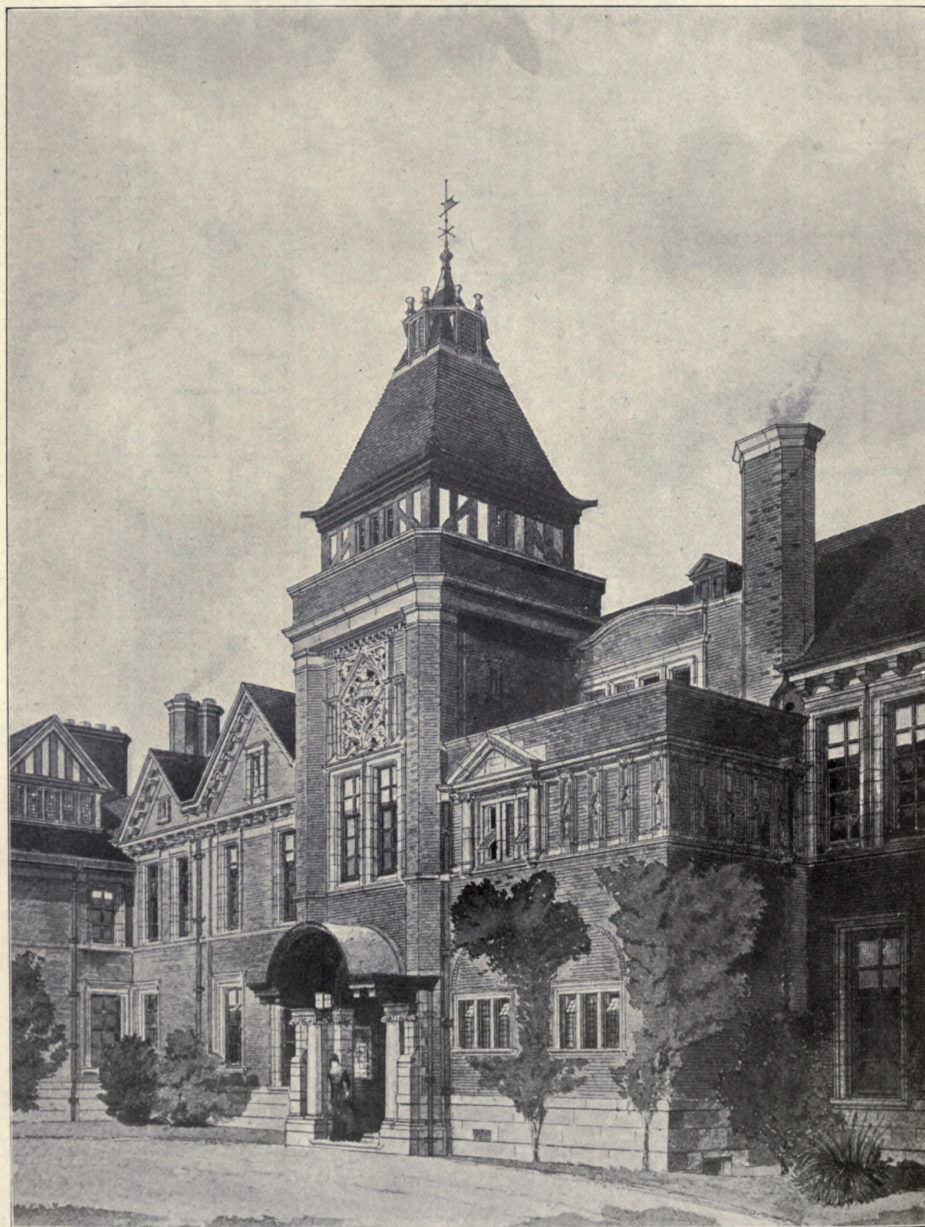
Moor Hall, Sutton Coldfield, Entrance Front, W. HENMAN AND T. COOPER, Architects. General Contractor: F. J. Briley, Hay Mills, Birmingham. Ornamental Leaded Lights: Harvey and Ashby, 49 John Bright Street, Birmingham.
