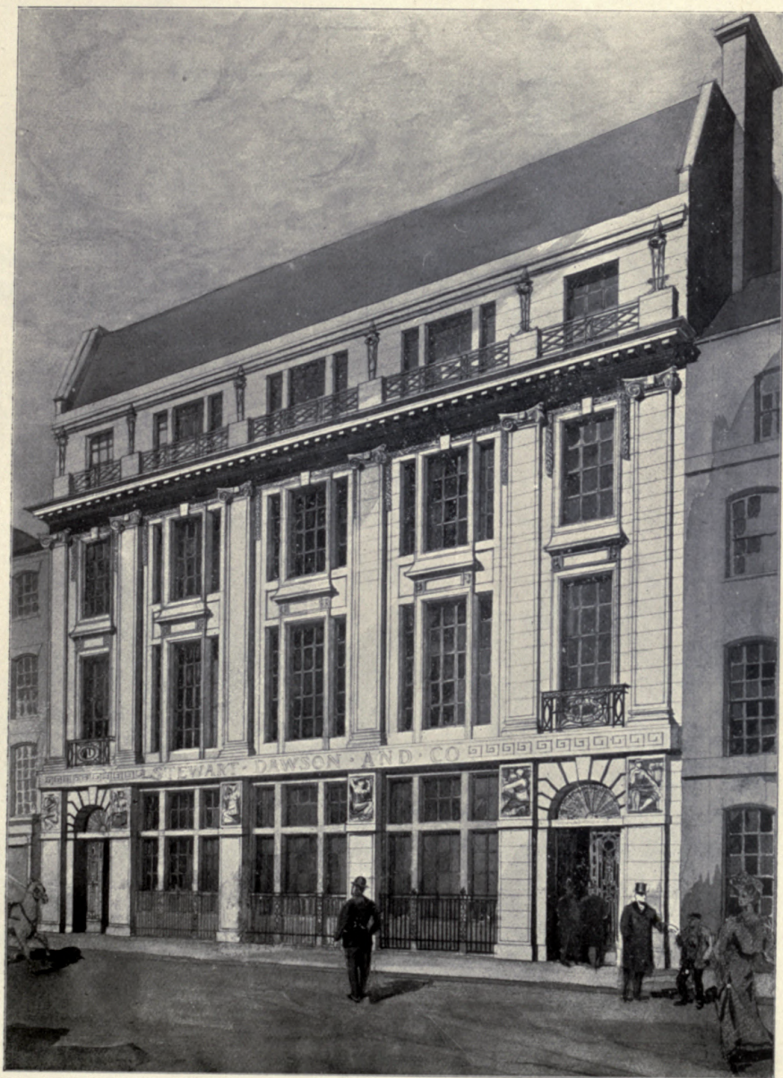
No. 19-21 Hatton Garden, London, NIVEN, WIGGLESWORTH AND FALKNER, Architects. General Contractor: J. Carmichael, 331 Trinity Road, Wandsworth, S.W. Constructional Engineers: Smith, Walker and Co., 37 Old Queen Street, E.C.
