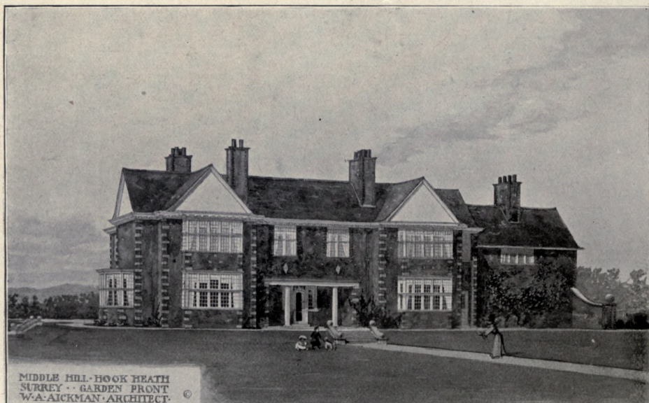
1518. Middle Hill, Hook Heath, Surrey, W. A. AICKMAN, Architect. (For Plans, see p. 123.)
