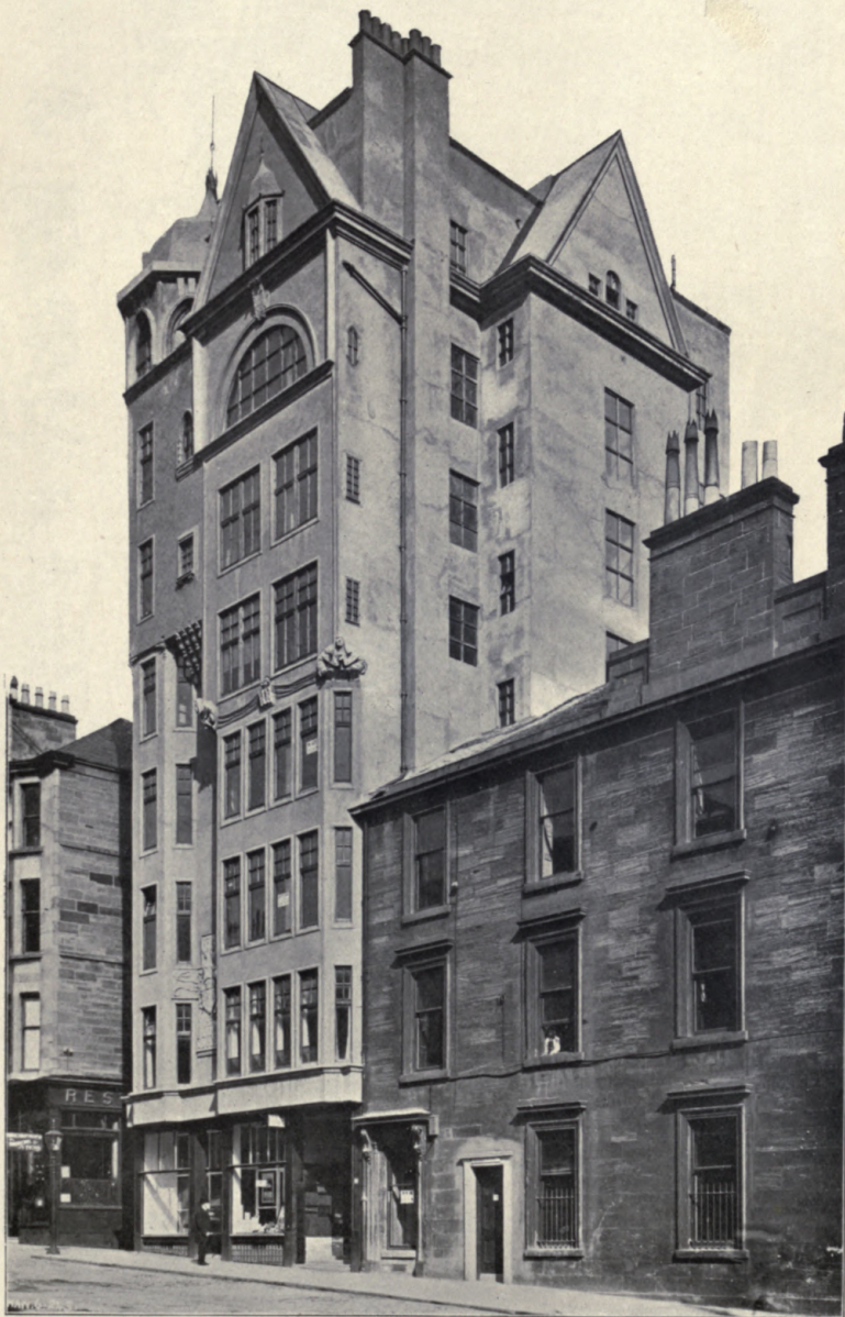
795. Lion Chambers, Hope Street, Glasgow, SALMON AND SON AND GILLESPIE, Architects. Ferro Concrete: The Yorkshire Hennebique Contracting Co., Ltd., Leeds. Joinery: Geo. Laird and Son, 10 Ann Street, Bridgeton, and 183 Bath Street, Glasgow. Elevators: A. and P. Stevens, 179 St. James' Road, Glasgow.
