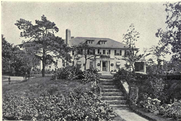
Residence of Richard E. Forrest, Cedarhurst, L.I., EWING AND CHAPPELL, Architects, New York.
