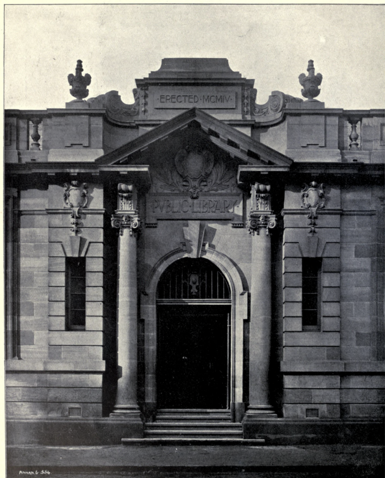
646. Springburn District Library, Principal Entrance, WILLIAM B. WHITIE, Architect. Masons, W. and J. Taylor, 183 Saracen Street, Possilpark.
