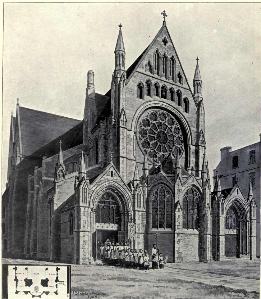
Church of St. John the Baptist, BROOK, SON AND ADKINS, Architects. Sculpture; H. H. Martyn and Co., High Street, Cheltenham.
