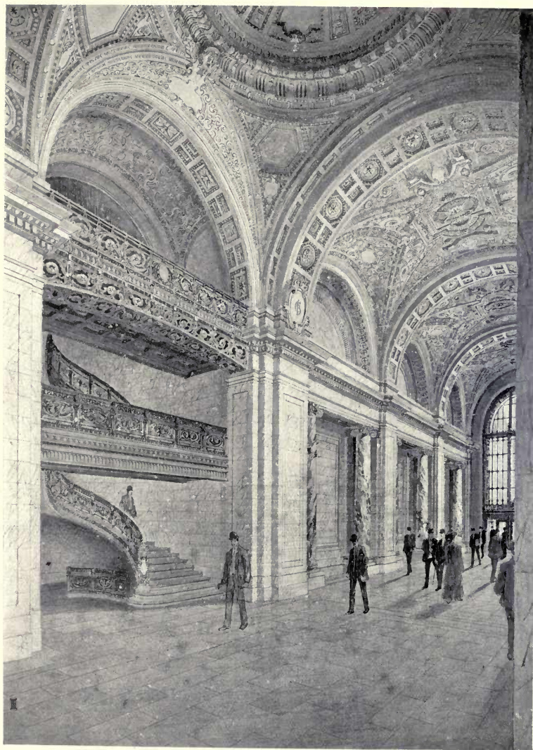
Interior, City Investing Building, FRANCIS H. KIMBALL, Architect, New York.
