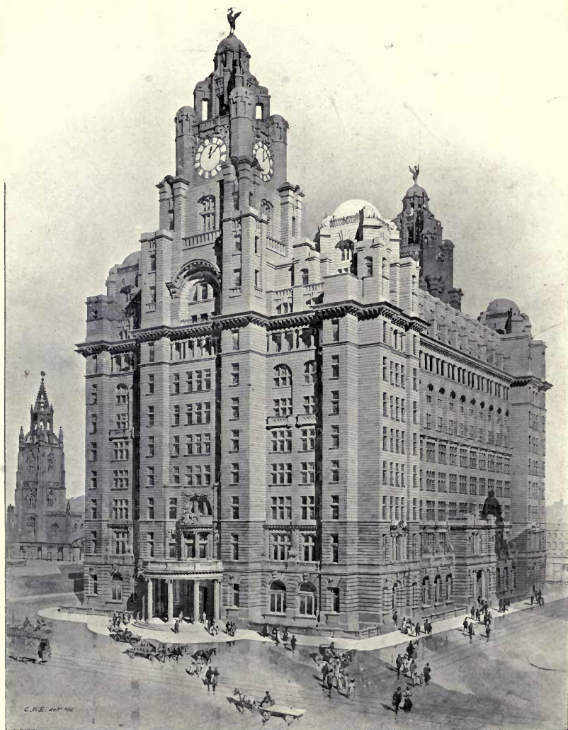
1703. New Chief Offices of the Royal Liver Friendly Society, Liverpool, WALTER A. THOMAS, Architect. Reinforced-Concrete: E. Nuttall and Co., Trafford Park, Manchester.
