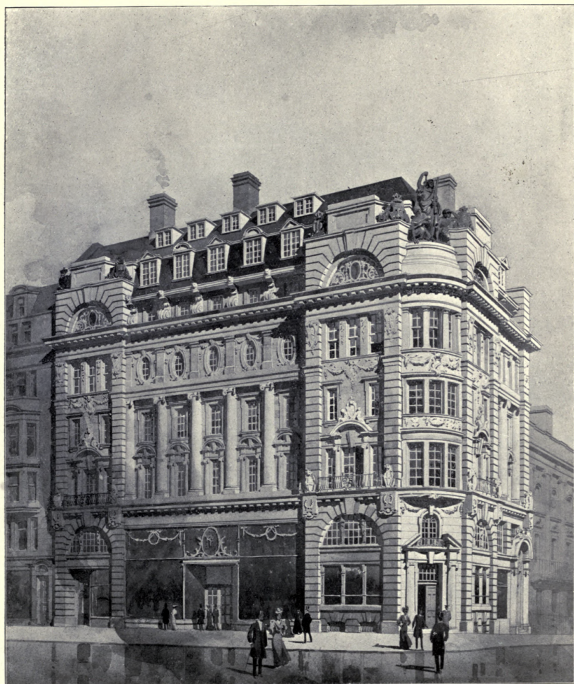
Norwich Union Life Insurance Society, Piccadilly, ERNEST RUNTZ AND FORD, Architects. Constructed of Solid Pentelikon Marble, from the Ancient Quarries, nr. Athens, of Marmor Ltd., 18 Finsbury Sq., E.C. Contractors: Patman and Fotheringham, 100-102 Theobald's Road, W.C., and Islington, N. Electric Lighting: Roger Dawson, Ltd., 1 Berners Street, W. Asphalte Work: Thomas Faldo and Co., Ltd., Effingham House, Arundel Street, Strand, W.C.
