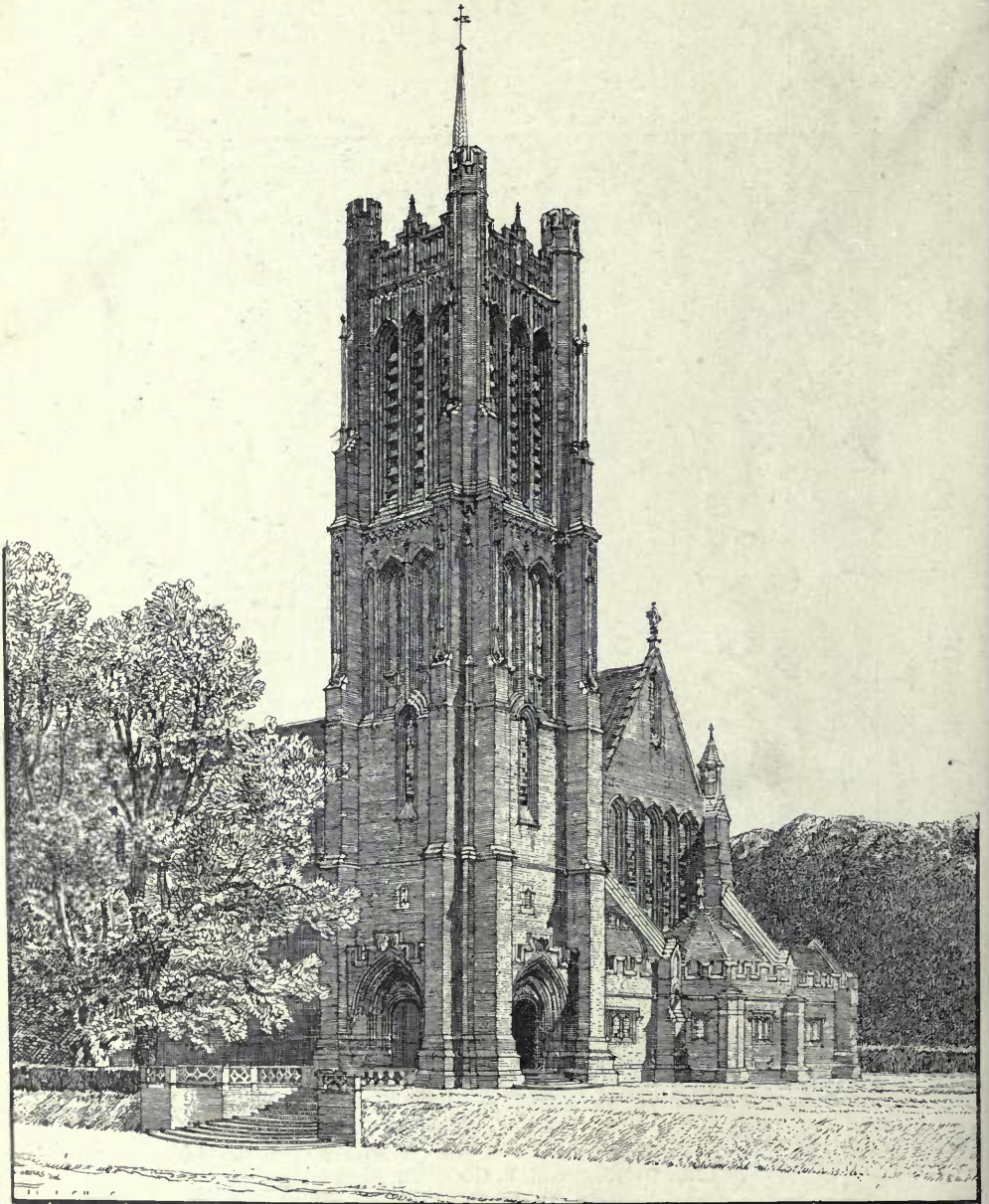
Christ Church, Sutton, Surrey, New Tower, Baptistry, and Northex, DOUGLAS G. ROUND, Architect.
