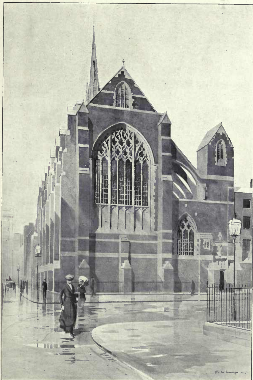
Church of the Annunciation, Old Quebec Street, W., South-east View, WALTER J. TAPPER, Architect.
