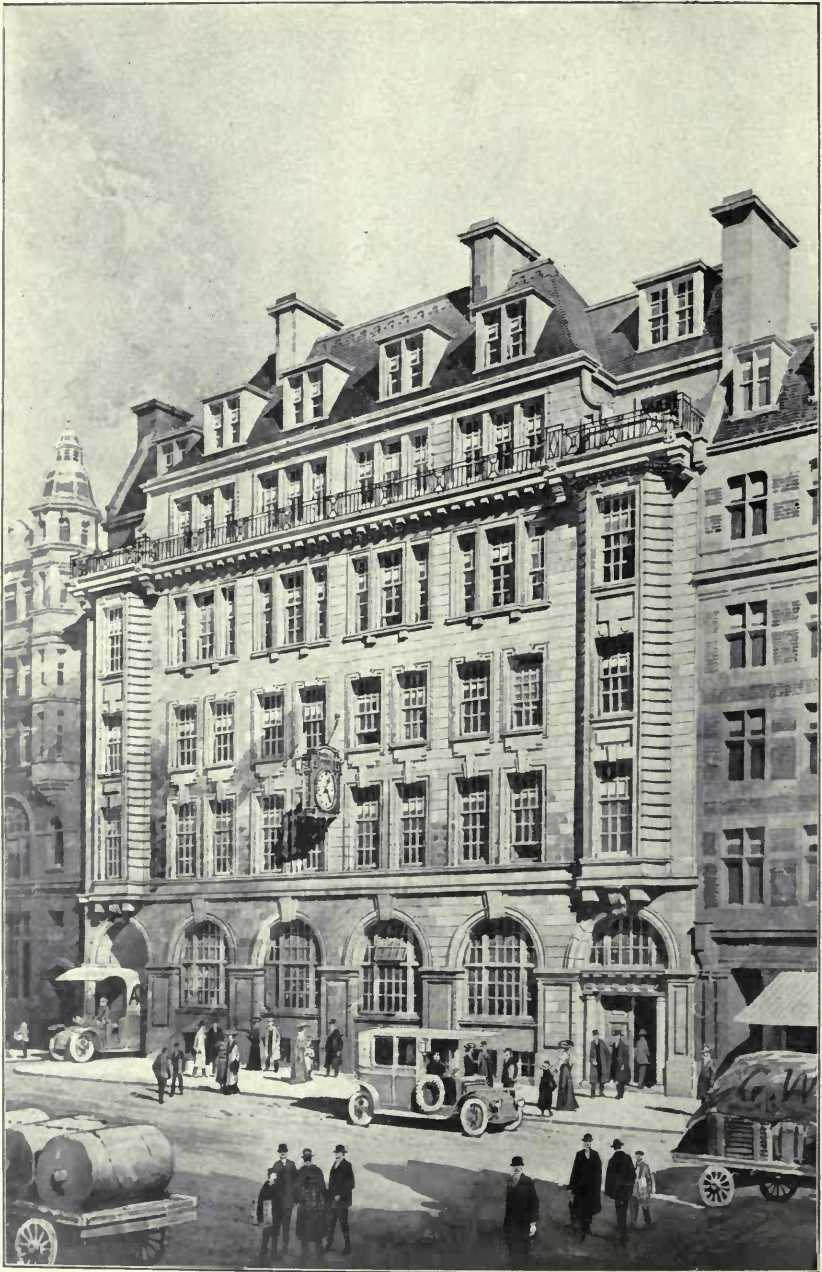
The Amalgamated Press New Premises, Farringdon Street, E.C.,
