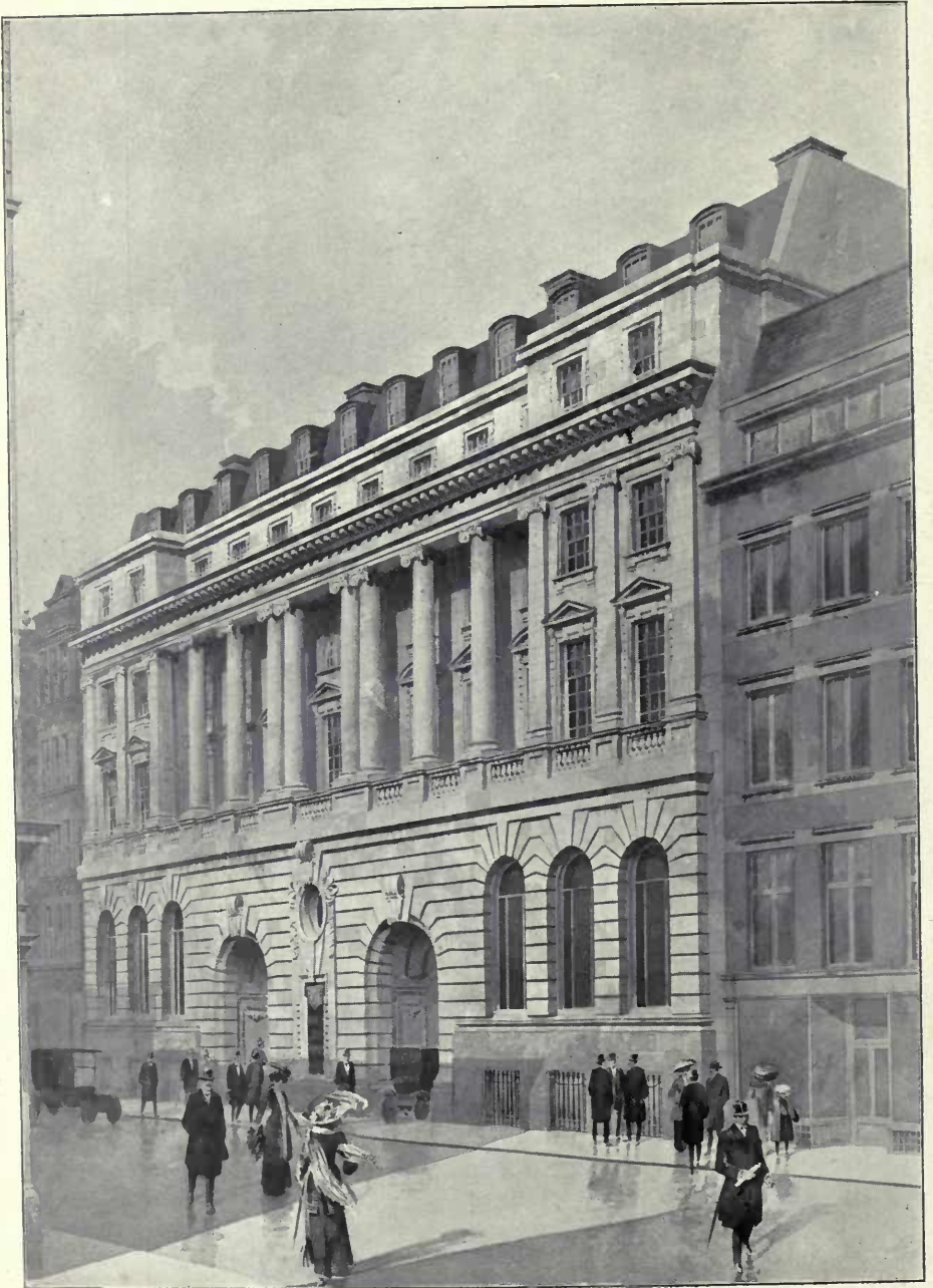
The New Premises for the Norwich Union Insurance Society, Ltd., Fleet Street, E.C., HOWELL AND BROOKS, Architects.
