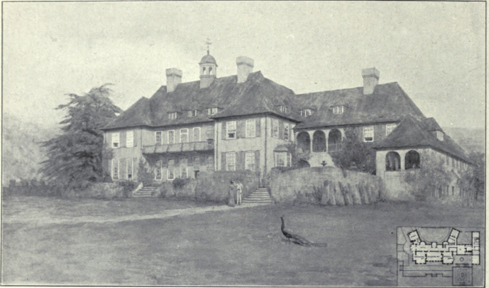
Ashford Chace, Petersfield, UNSWORTH, SON AND TRIGGS, Architects.
