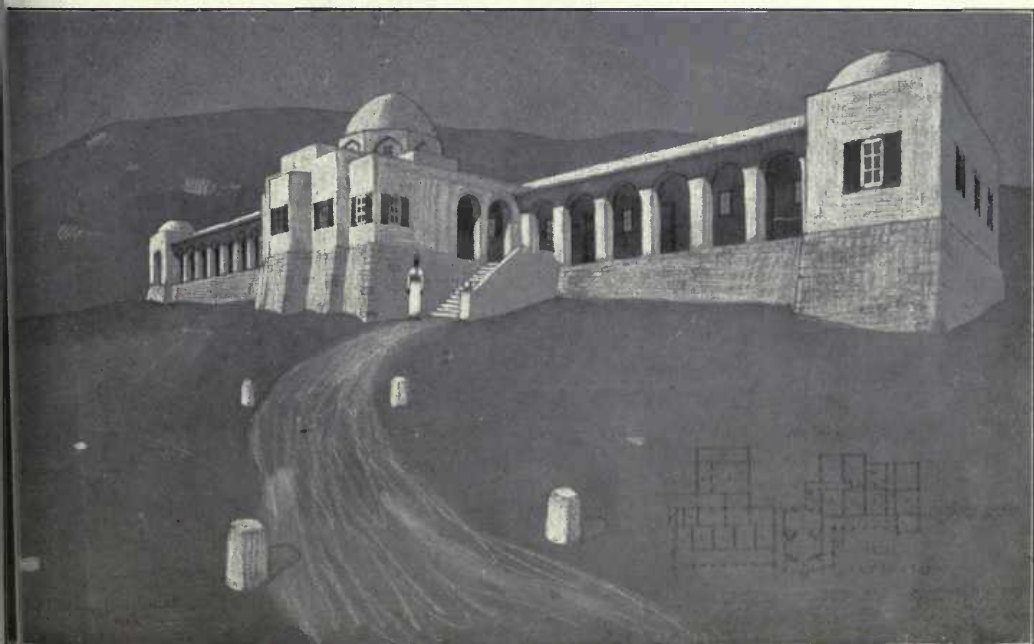
House at El-Assasif, near Luxor, Egypt, W. J. PALMER JONES, Architect.
