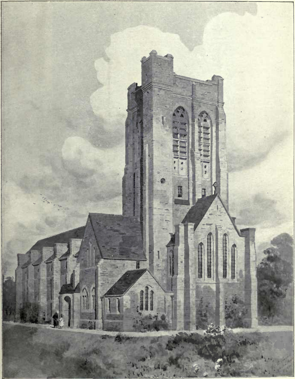
1609. Church of St. Ninian, Douglas, Isle of Man, WILLIAM D. CARÖE, M.A., Architect.
