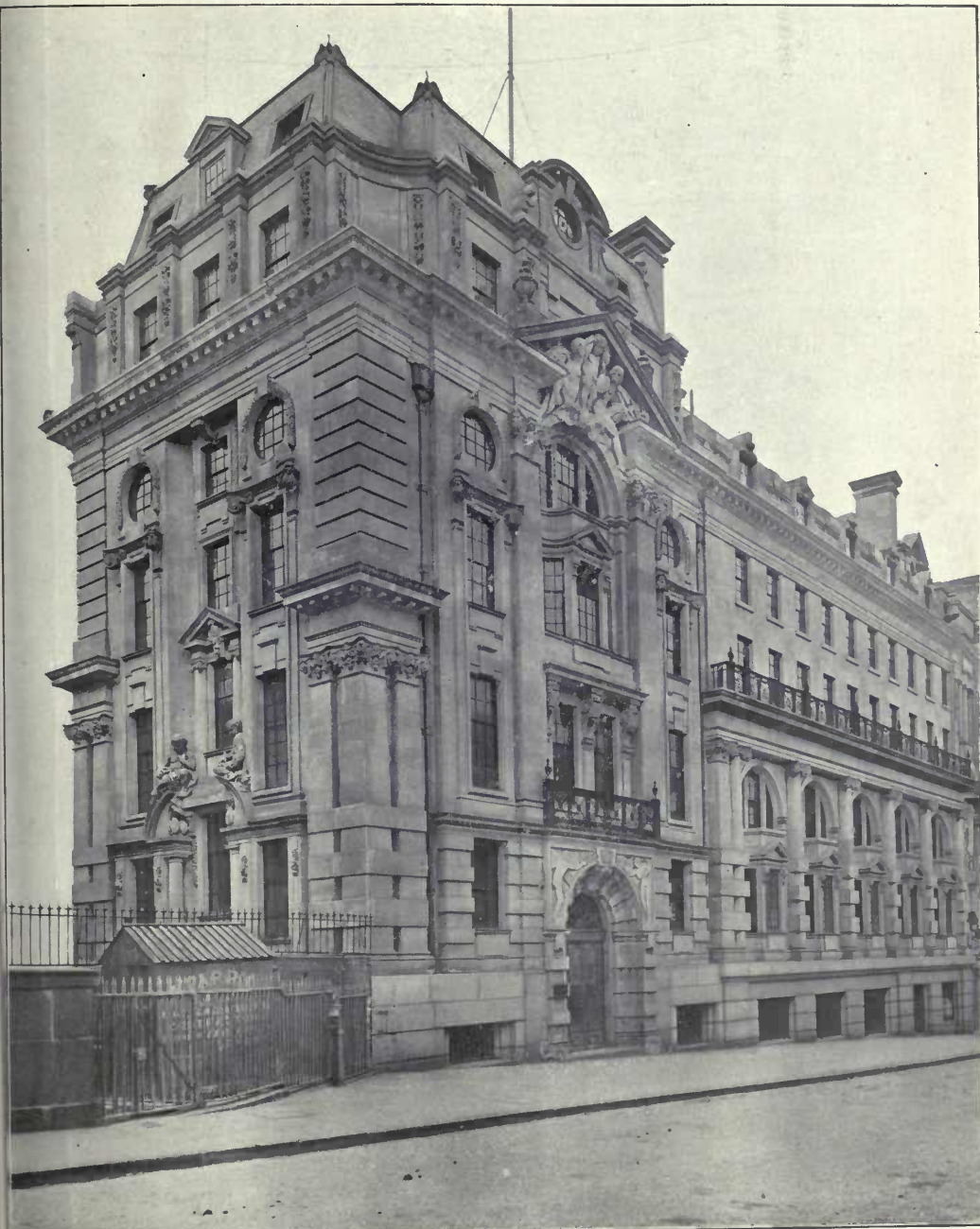
"Thames House," Queen Street Place, London, E.C., T. E. COLLCUTT and HAMP, Architects. RICHARD GARBE, Sculptor.
