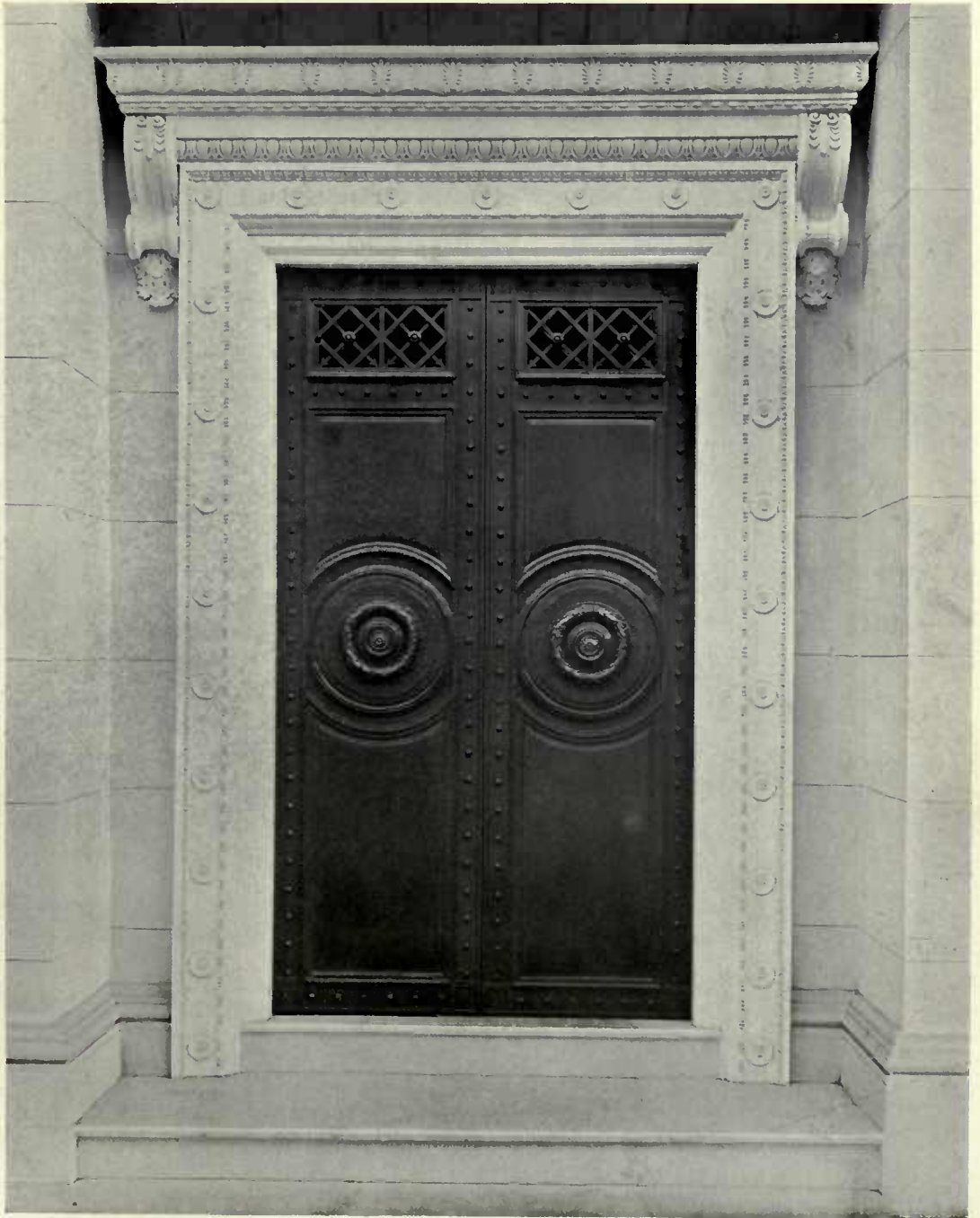
Doorway, Central Heating Pavilion.
