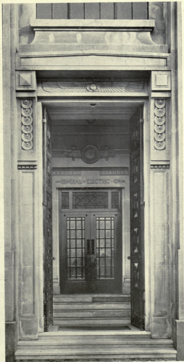
GENERAL ELECTRIC CO., WITTON, BIRMINGHAM. ADMINISTRATION OFFICES : MAIN ENTRANCE. WALLIS, GILBERT AND PARTNERS, ARCHITECTS.
