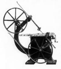
The cuts of the band saw shown on this page show a new machine that is a decided innovation from the common type of machines. The machine is designed to overcome the difficulties and inconveniences incident to the tiltingtable machines; and on this machine the table is always level whether doing square or angle sawing, regardless of the angle
