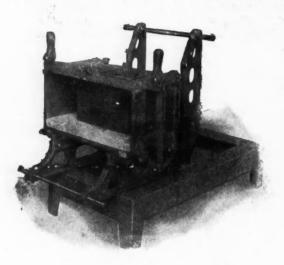
ated by inexperienced labor. It can produce a larger amount of better blocks per day than any machine on the market. Either wood\* or iron pallets may be used. It is built low down, so that a man working it stands in a natural position.
