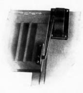
and forms of windows, working to particular advantage on bay, mullion, corner and angle, yet requires no lubricating, and when once installed no further attention is required to keep it in order. The device prevents the blinds from blowing off the hinges, at the same time being easily detached for painting or other purposes. It does
