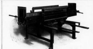
Machine with extension to make all long stone up to 5 ft.; 6 in. long
