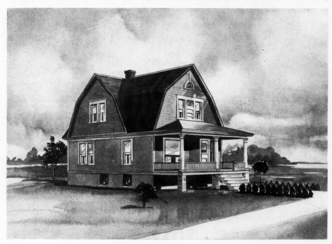
water shed. The slope is not lost because the odd spaces are uses for clothes closets and the stairway. A roof of this kind may be built almost as easily as any other and it certainly offers considerable advantage in the way of extra room.
