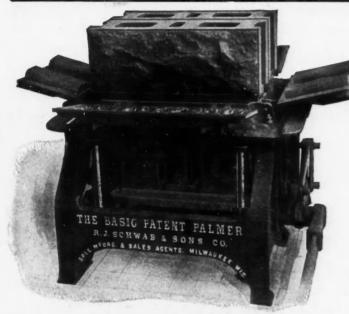
Showing Machine Open With Two Blocks Made at Once Ready for Removal
