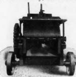
of the American Mixer. Its superiority is too evident. Revolving plows inside the drum do the work.
