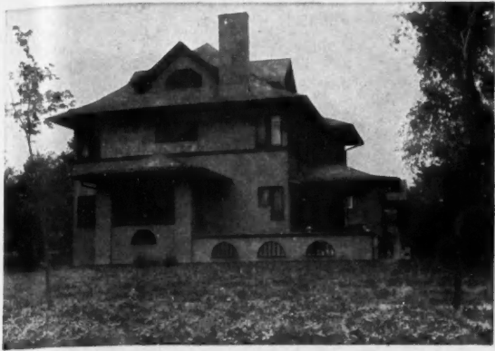
HEATED WITH A HESS STEEL FURNACE
