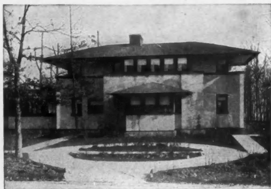
HEATED WITH A HESS STEEL FURNACE
