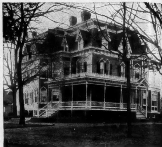
HEATED WITH A HESS STEEL FURNACE
