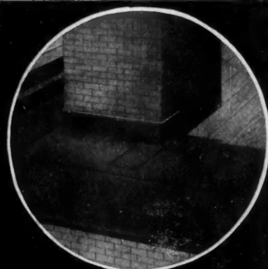
Flashing—Roof Book, page 13, tells how to make it.
