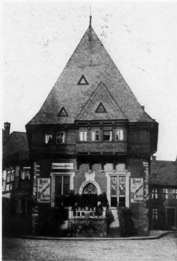
"Some of the Tallest Buildings Hold out in Front Like a Shield, Little Duplicates of Themselves"
