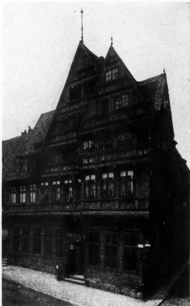
"Surmounted by Three Triangles, Each Story Projecting Farther Outward Than the One Below to Show Its Fine Wood Carving"
