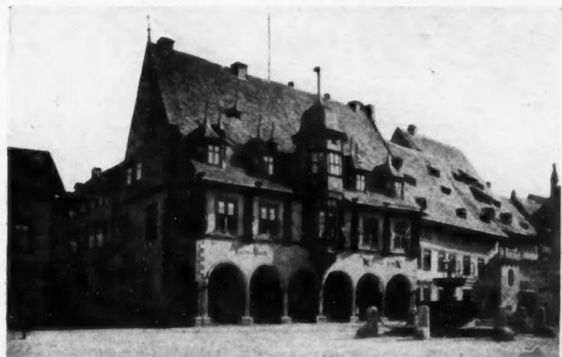
"Where the Roof Windows Take the Form of Towers of Varying Sizes"
