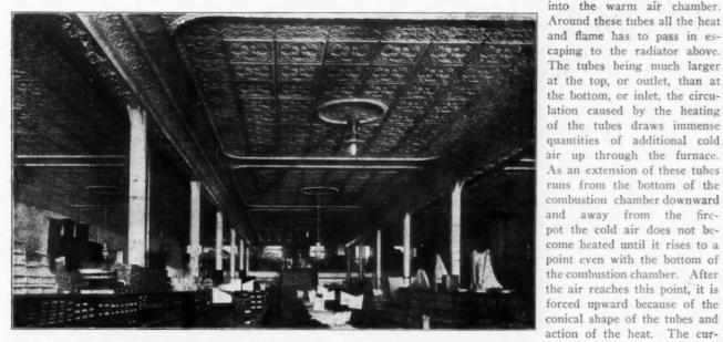
their slight increase in cost over lath and plaster. Closely joined, or interlocked, so as to make them easy and economical to install, they present an almost air-tight surface and being incombustible, they tend to greatly protect floors and woodwork in cases of fire, and have many times, by preventing the spread of flames until the arrival of the fire department, saved buildings from destruction. Being of
