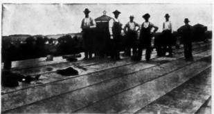
This view shows Three Ply "Ford's Calvanized Rubber Roofing being laid on the New Hampton Auditorium, New Hampton, Is The cut below shows the completed structure.
