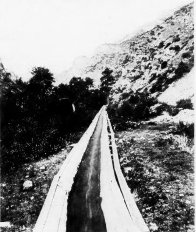
V Shaped Timber Flume, Sheridan County, Wyoming
