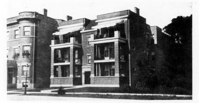
No. 4. A new six-flat building on Sheridan Road. It represents the best and most fashionable type of flat construction. There are eight rooms and two bath rooms in each flat. Four solid brick walls extend through from front to back, and the construction is what is termed "slow burning." At the left is another six-flat building about two years older. Few private porches were built up to two years ago.
