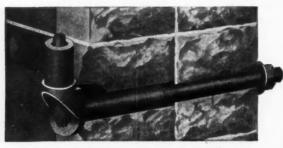
most effectively solved, your attention is called to the illustration, which shows a fire shutter hinge device, and the manner in which it is placed in a wall.
