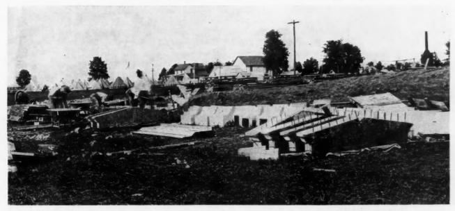
Fig. 2. Door and Window Caps, Decorations, Etc., Molded Separately-Notice the Reinforcing Metal
