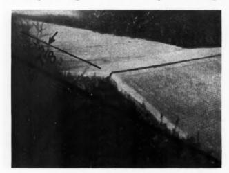
from 8 degrees below zero to 93 degrees above, or 101 degrees variation, without the least injury. Nevertheless, it expanded and cracked last May, when the temperature did not vary more than 30 degrees in 24 hours, and when freezing was entirely out of the question. Upon investigation, it was found that the excessive rains had caused the drains under the walk to become clogged, hence expansion by moisture was the sole cause of the trouble.
