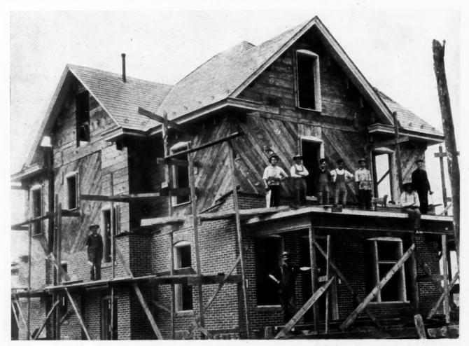
House of Brick Veneer Construction Being Erected By C. G. Burkett at Warriorsmark, Pa.
