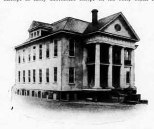
composed of Cortright metal shingles, the embossed design of which is very pleasing to the eye and serves to attract attention to the building, although this had no consideration in the selection of the material—the principal feature considered that led to their selection being the wear; the manufacturers claim that they will last as long as the building itself, and if
