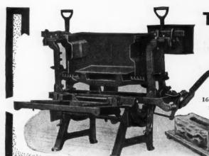
With the "Oliver" all changes for making all the different sizes of blocks are made without the use of a wrench. pick out one set of plates and place in another. The "Oliver" makes blocks running every inch from 2" to 24" in length, and from 4" to 12" in width; also 4", 6", and 8" height blocks.
