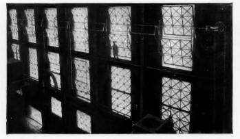
Four lines of sash, each eight feet high, controlled with one gear.
