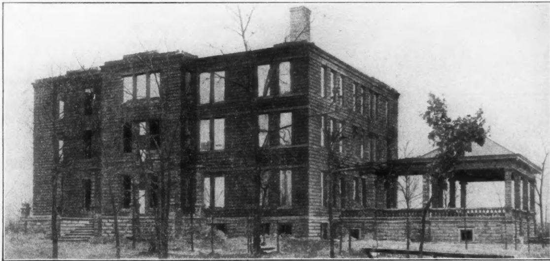
After Fire, Nothing Left but Walls of HERCULES Stone.
