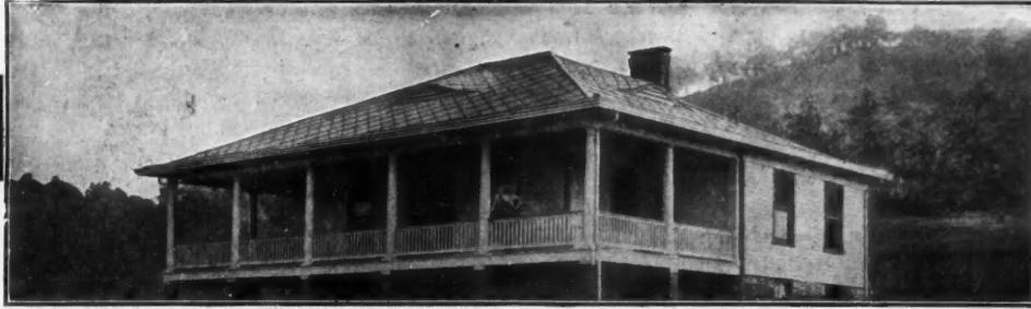
Asbestos "Century" Shingle Roof—Dayton Gun Club, Dayton, Ky.; William Lampe, Newport, Ky., Architect; R. L. Brown, Covington, Contractor
