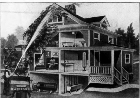
Lay-out of Modern Water Supply System Installed in Residence
