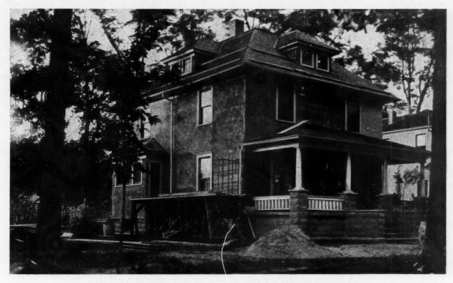
House at Niles with "Scratch" Coat Partially on. Note Furring Strips and Lath
