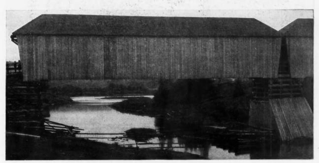
Fig. 3. Modern Wooden Bridge, Covered to Protect the Timbers
