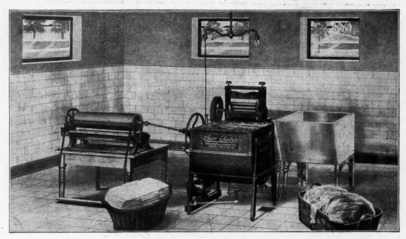
The "THOR" Electric Home Laundry Machines are on the cylinder principle just like the large laundry machines but are built especially for home use. Made in two sizes. Will last a lifetime. Write for Booklet Write for Booklet.
