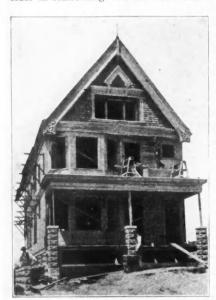
care has been taken as to the angle at which it rests to the building, so shifting the weight that a thousand pounds is easily carried at the extreme outward end of the bracket, making a scaffold as safe for the carpenter to work on as though he were upon the ground.
