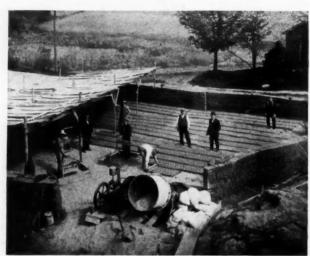
Method of Placing Product for Curing.
