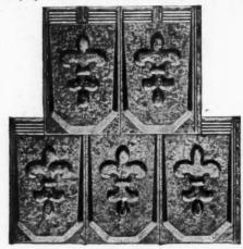
Neverleak metal shingles no solder is required, and there are no exposed nails. The accompanying illustration shows one of the designs of this metal shingle. It has been said that a roof should be more than a mere protection; it should ornament and increase the value of the building to which it is applied. There is no question regarding the artistic and attractive qualities of the Neverleak metal shingle.
