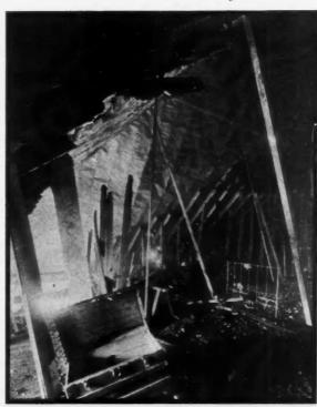
View from Within—Building Shown Above. The Wooden Props Were Put In After the Fire to Keep the Tin From Collapsing In The Wind
