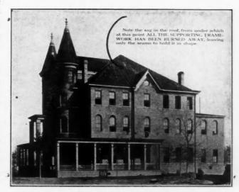
Tin Roof that Kept the Fire Inside, Itself Holding Fast After Supporting Timbers Had Burned Away
