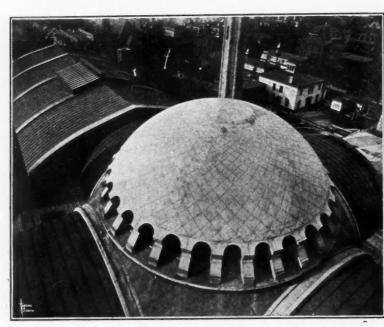
Tin Roofing for Curved Surfaces - Square Sheets Laid Diamond Shape
