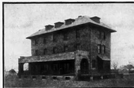
Asbestos "Century" Shingle Roof—Residence of J. H. Briggs, Sea Gate, Coney Island, Brooklyn, New York; Squires & Wynkoop, New York, Architects: P. J. Van Note, Brooklyn, Contractor.
