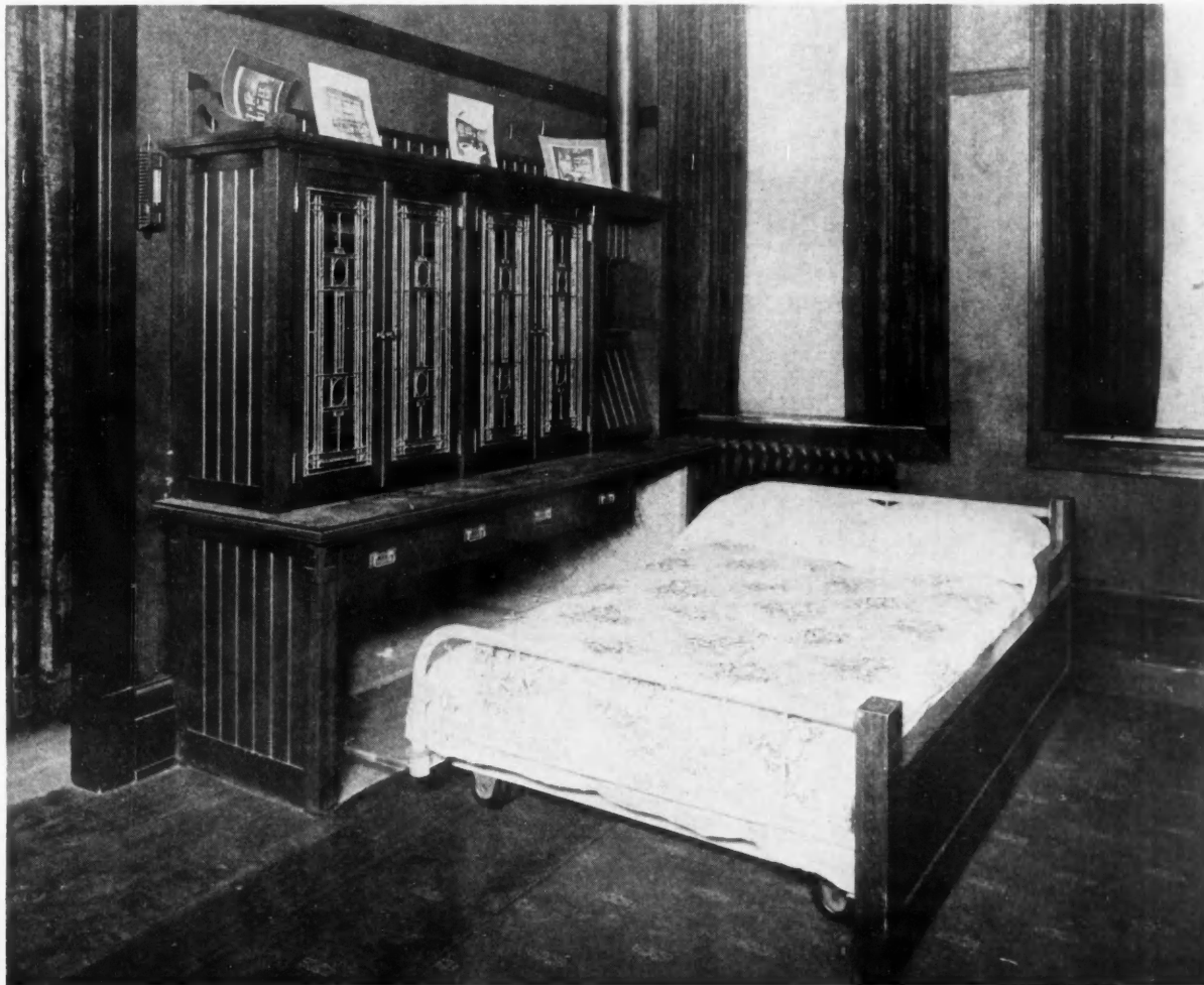
This Bed Goes in Sidewise—A Cupboard or Seat in Adjoining Room Covers the Bed Recess
