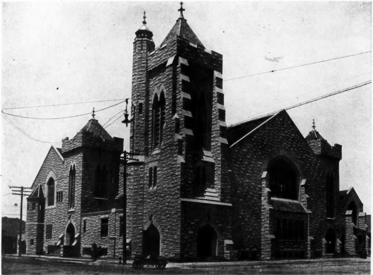
Methodist Church, Long Beach, Cal. Artificial White Granite, Made by H. H. Hamilton.
