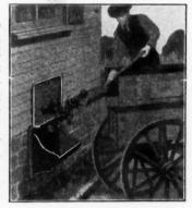
conditions, and will admit of ample light to the basement. These chutes are constructed so that during the heated term the "rubber glass" can be removed and a screen inserted in its stead, allowing pure ventilation.
