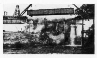
Fig. 2. Dynamiting the Old Trestle to Make Way for the Girder
