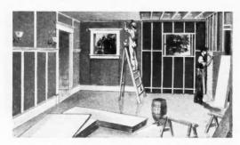
Nailing Beaver Board to the Walls and Ceiling of a New Room.
