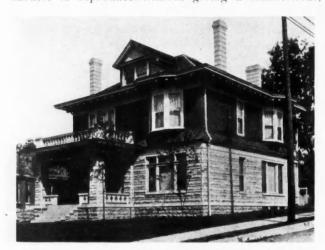
Rough Finished Blocks in Two Widths in Combination with Shingles
