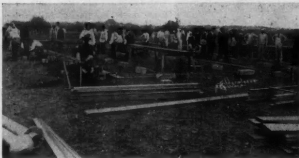
8:30 A. M.—Material and Men Arrive and Work Starts
