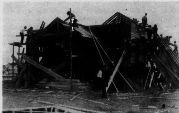
Noon—Progress Made by 50 Carpenters
