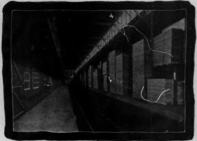
Interior View Loading Platform
