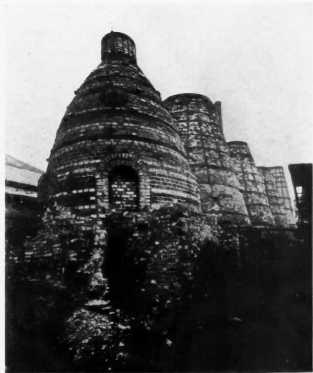
Fig. 6. PORTLAND CEMENT KILNS OVER SIXTY YEARS OLD. Built in 1848 at Northfleet, Kent, England, by William Aspdin, Son of Joseph Aspdin, Inventor of Portland Cement. Kilns of Upright or Dome Type, with Intermittent Draft.
