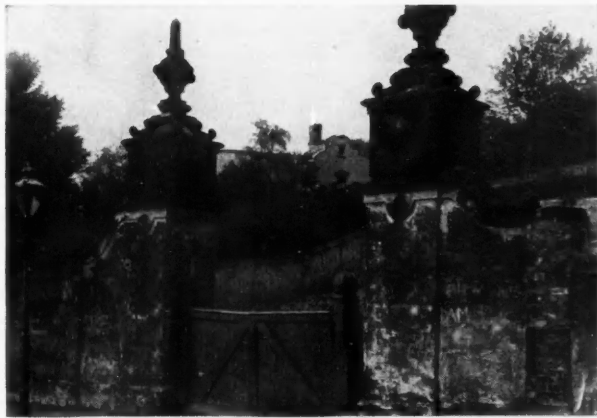
Fig. 4. HOW "PORTLAND HALL" LOOKS TODAY. Structure in Background, now used as a Private Residence, is only Portion of "Hall" that was Completed. The Cement Stucco on the Brick Walls Around the Grounds, and on the Gate-Posts, is Probably the Oldest Example Extant of the Ornamental Use of Portland Cement.
