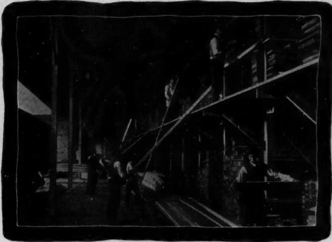
Finishing Lumber Shed No. 2
