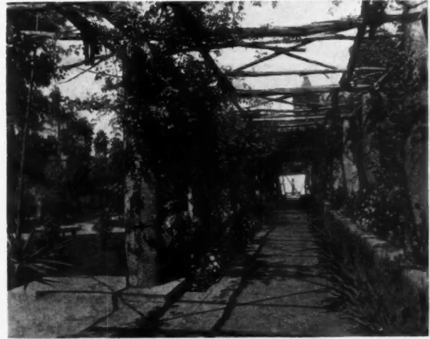
Pergola with Cement Plastered Pillars and Rustic Canopy
