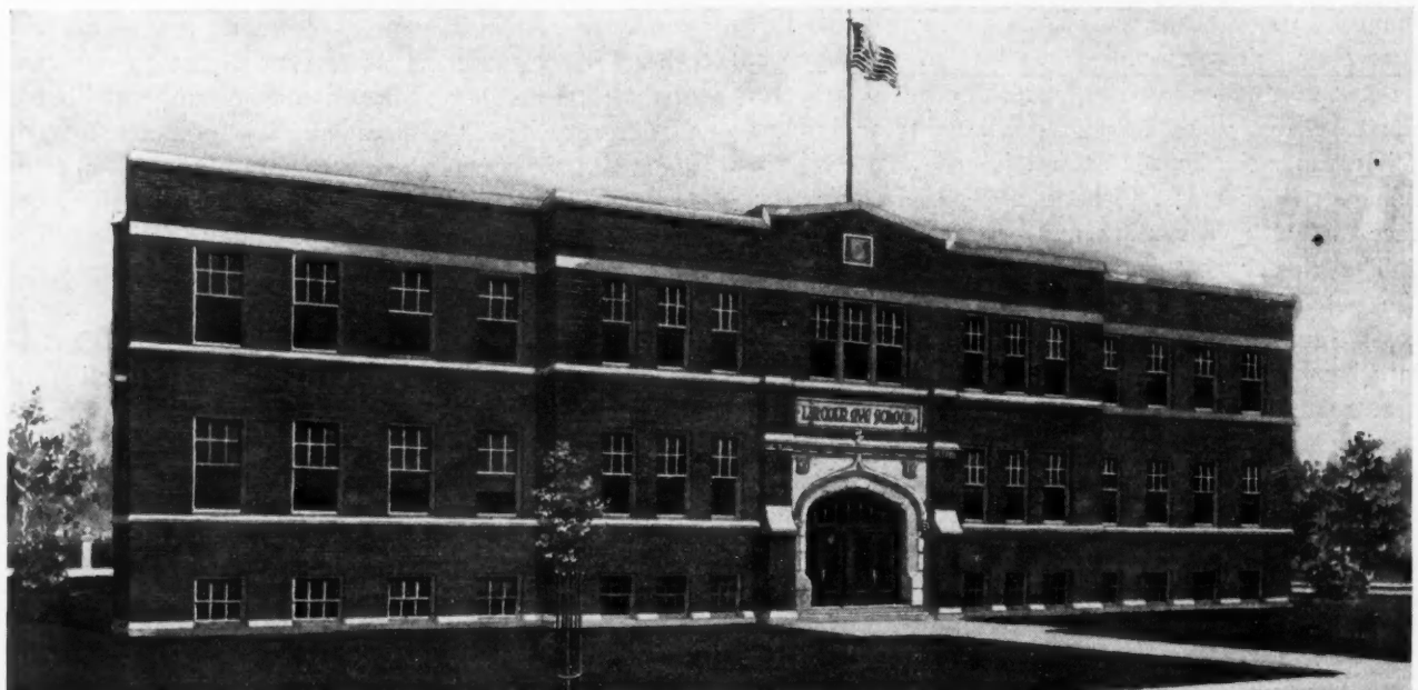
New Lincoln Ave. School, Dolton, Ill.; Architect, G. W. Ashby, Chicago
