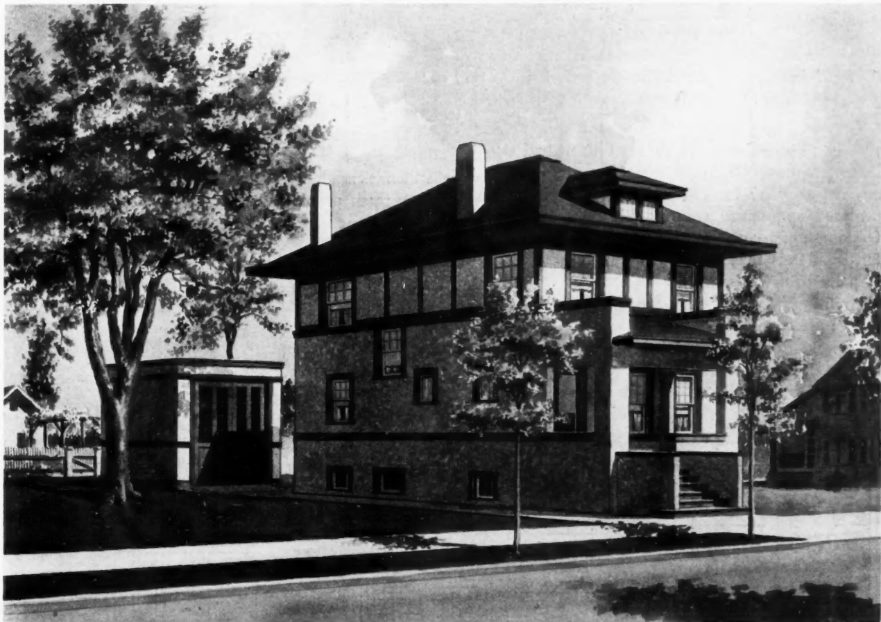
Up-to-Date Stucco House Designed for Mr. J. A. Beckwith of Chicago COMPLETE WORKING PLANS FOR THIS HOUSE ARE PRESENTED ON THE 7 PAGES FOLLOWING
