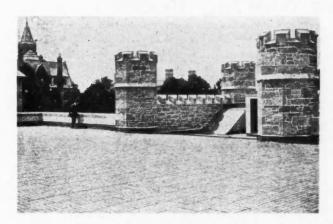
Flat Slate Roof on Gymnasium of Bryn Mawr College. Slate is cut three inches square and laid in asphalt.
