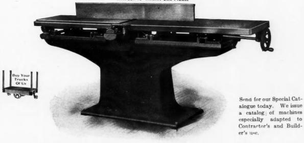
Used for Planing, Jointing, Shaping, Matching, Rabbeting, Grooving, Chamfering, Beading and Making Mouldings.
