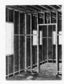
Room ready for Beaver Board construction, studs evenly spaced and headers in correct position to suit panel designs adopted
