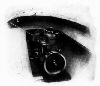
Showing Proper Installation of Motor in Boat
