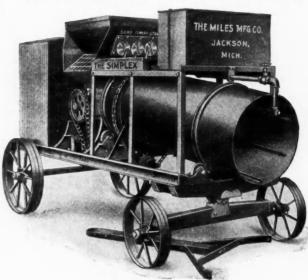
for handling sand, gravel or stone. These different materials are all conveyed into the mixing drum absolutely continuously, which makes a fairly thorough mix before the materials ever start on their rolling course through the mixing
