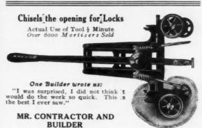
Our patent double edge, side cutting chisel can cut more wood, four times more rapidly and 100% less exertion than any boring bit.
