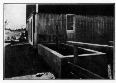
Concrete Tank with Removable Tank Heater
