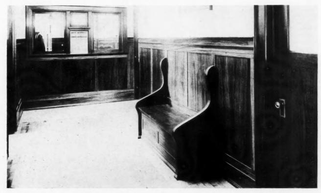
Paneling of Rotary Cut Red Gum—This Finish Produced with one Coat Linseed Oil Followed by a Coat of Shellac and Two Coats of Varnish, the Last one Being Rubbed to Dull Finish
