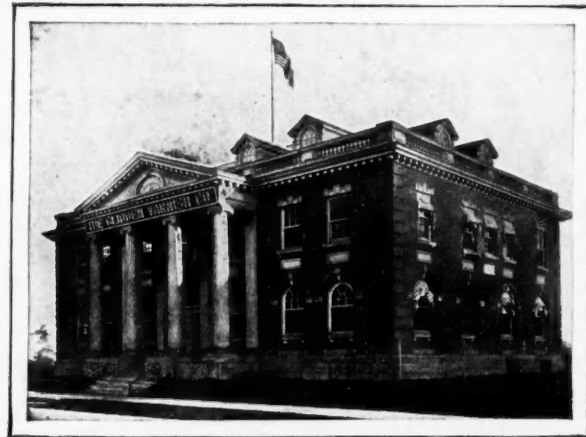
Administration Building, Glidden Varnish Co.
