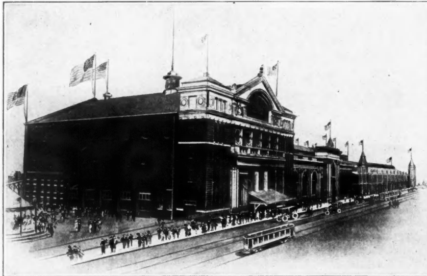
Exposition Hall, Duquesne Way, Pittsburgh, Pa. Where the First Pittsburgh Cement Show will be held, December 12-18, 1912
