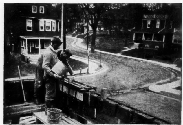
Making ready to insert the floor beams.
