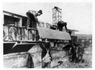
Swinging Form Plates at Nanticoke, Pa. Note Tie-bars Projecting to Form Support for Scaffold Planks
