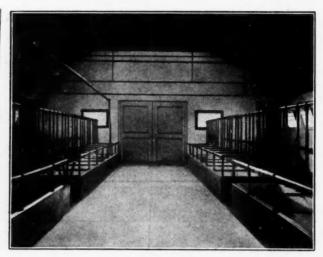
Interior of Concrete Cow-Stable, Built by Van Guilder Hollow-Wall Machine
