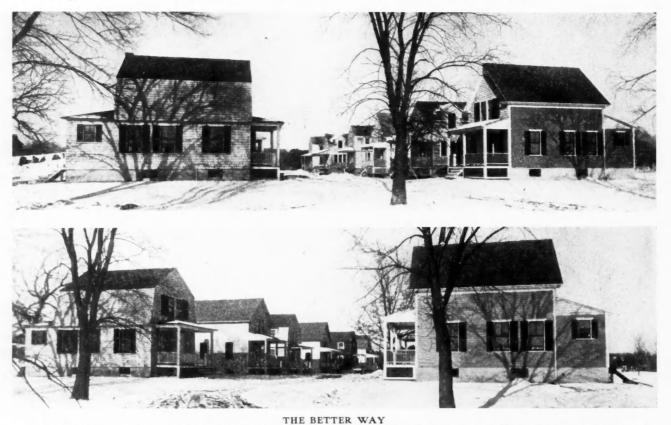
Two Views of Street of Twelve Houses Built at Framingham, Mass., by the Framingham Associates. Each House Contains Five Rooms and a Bath. Concrete Cellar and Foundation Walls, Furnace, Well Built and Good Plumbing. Size of Each Lot 50 ft. by 87½ ft. Cost of House and Lot, About \$1,700. Sells for About \$1,900. Could be Rented for \$15 Per Month
