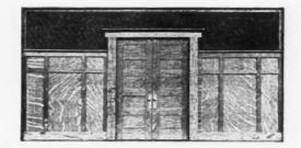
**CAL-CO-CRAFT** is a reproduction of wood grain (taken from the actual wood), transferred to paper—hung like any wall paper and paneled off with simple mouldings — note cut above.
