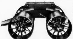
The standard four wheel truck shown is perfect in strength, weight and durability. It will carry 40 tons. These trucks have 3 inch carbon steel axles and either cast iron or wood bolster as desired. The rear axle has special bracing.
