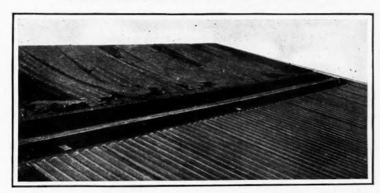
THE above photograph shows a roof specially constructed of black steel sheets (no coating of any character). The upper portion displays a corrugated roof of ordinary steel, which is almost decomposed. The lower portion shows a roof of "COPMETL" in almost as GOOD CONDITION AS THE DAY IT WAS LAID. Both sections were laid simultaneously and were exposed to the atmosphere for the same period. Both portions are of No. 27 Standard Gauge.
