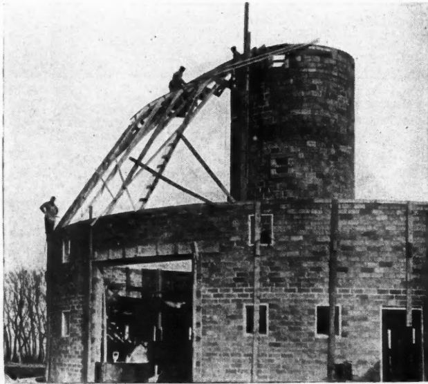
Framing the Rafter Trusses
