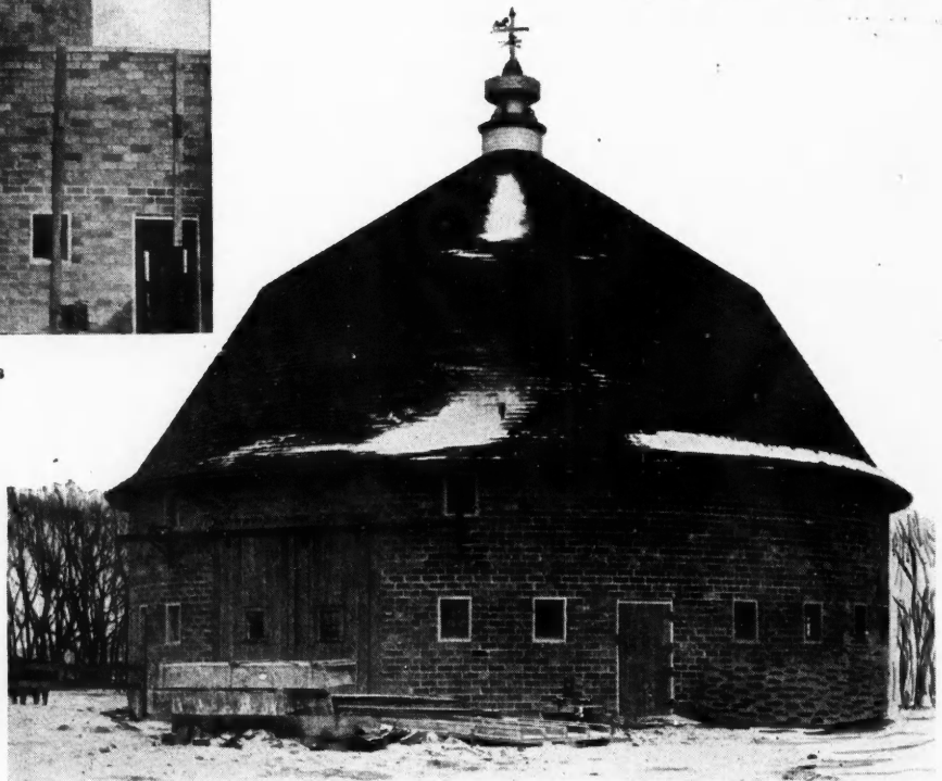
View of Completed Barn—Planned and Built of Denson Tile by the Northern Construction Co., Mason City, Ia.
