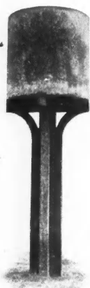
Graceful Concrete Tank
