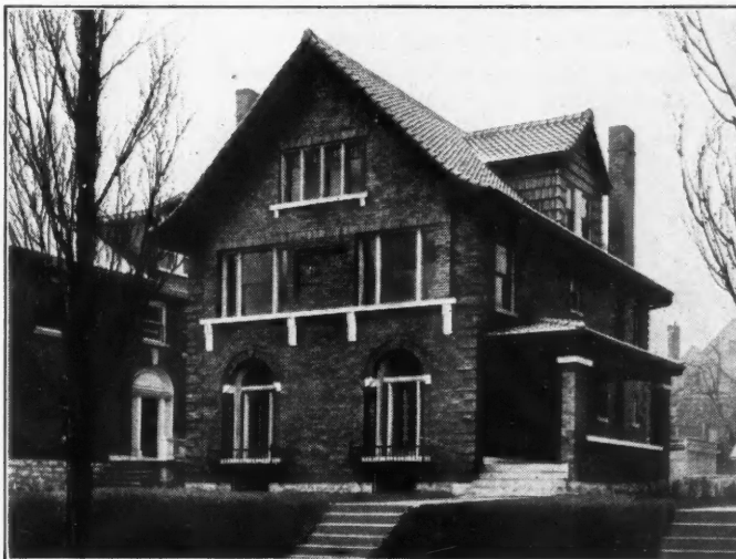
This House, Built of Hy-tex Brick, Cost $9,875; Only $430 More Than for Clapboards
