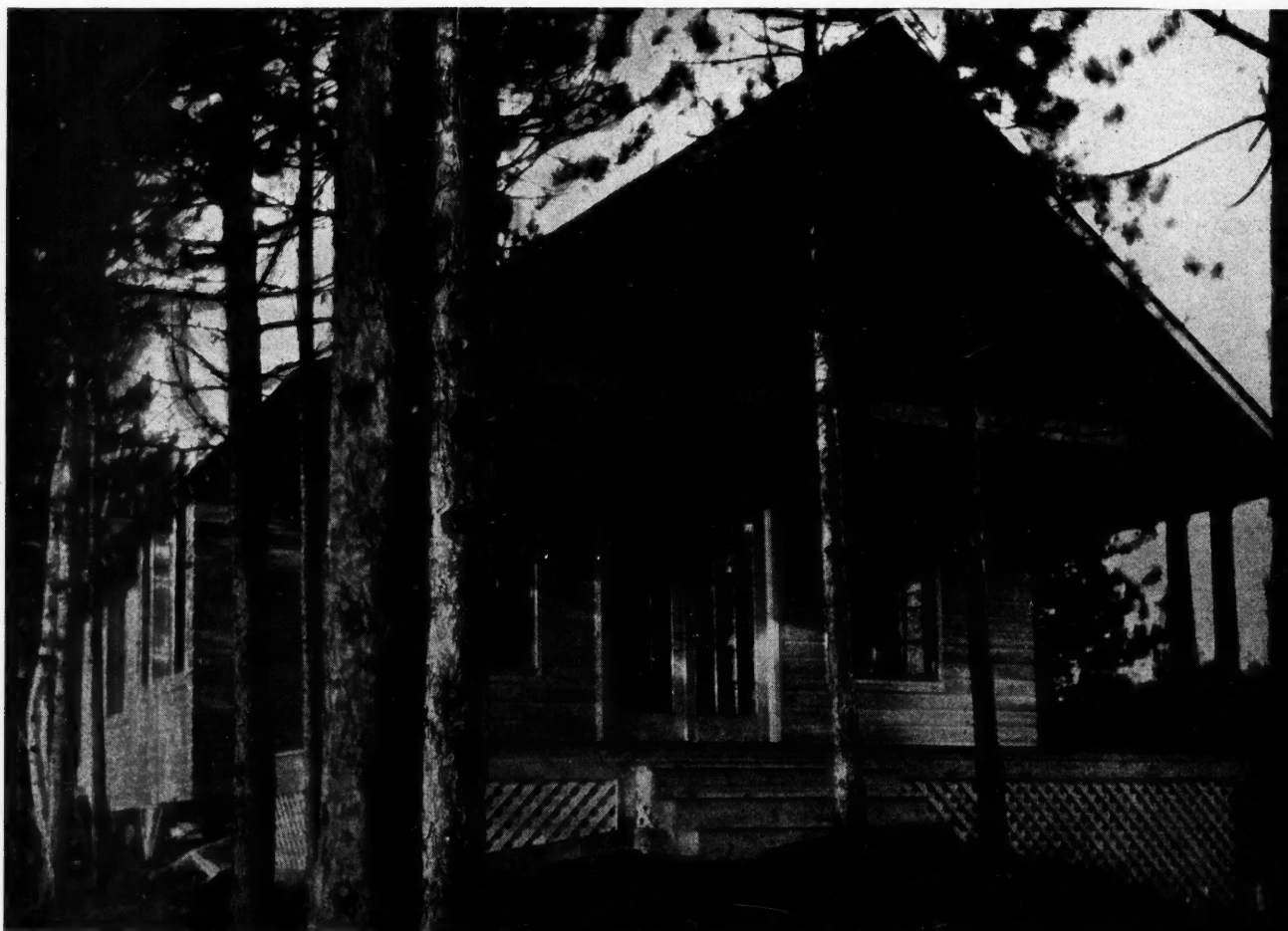
This Cottage has four Rooms besides the Sleeping Loft and the Two Big Porches. It has been pronounced one of the best designed small camps in the New York Mountains. Cost, Complete $1,300
