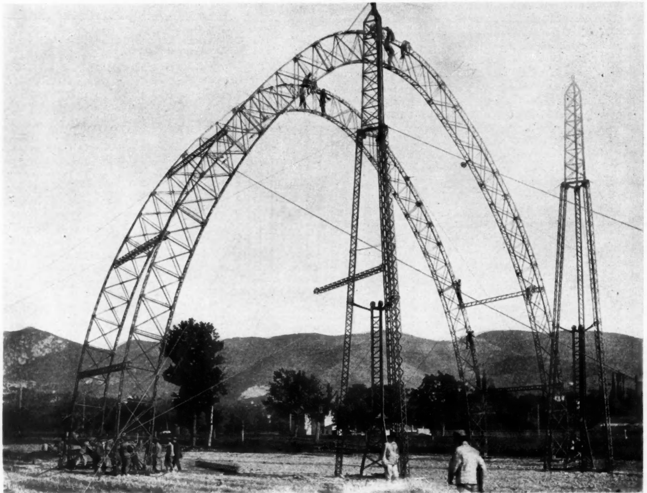
Italian Army Engineers Erecting Light Framework for Dirigible Balloon Hangar
