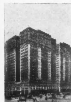
Hudson River Terminal Bldg., N. Y.
