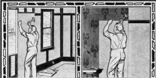
Nailing Beaver Board to studding of a new room.
