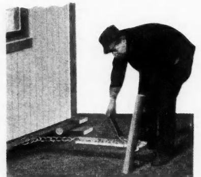
Jack Being Used to Move a Building
