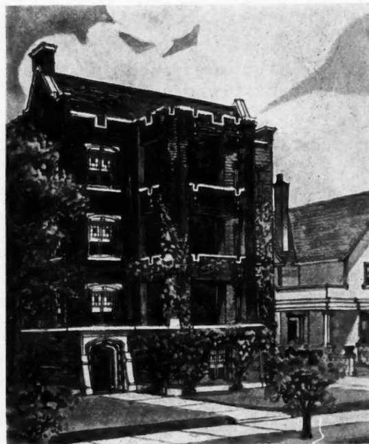
One of the Beautiful Chicago Apartment Buildings Recently Floor Finished With Triple "A" Machines.
