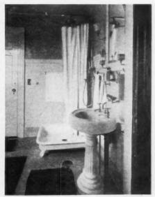
Modern Bathroom Finished in White, the Floor and Wainscoting in Tile—Oilcloth Waterproof Paper Covers Upper Walls and Ceiling
