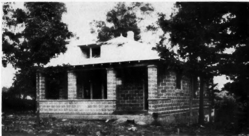
Neat 5-Room Concrete Cottage in Course of Building
