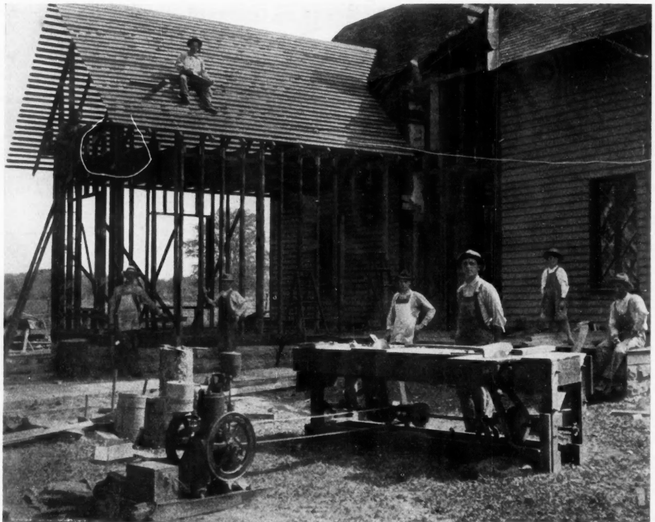
Contractor Henderson and His Gang on a Recent Remodeling Job. His Gas Driven Combination Portable Woodworker Does All the Heavy Work and a Good Deal Besides
