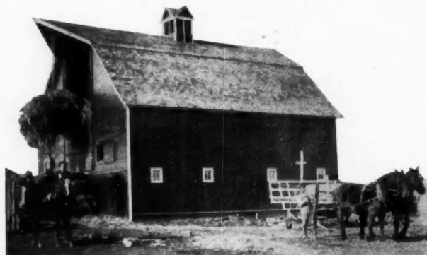
Well Designed Barn at Greeley, Nebr.
