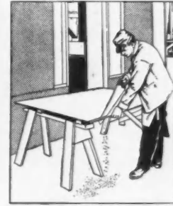
5—SAWING Use a fine, panel saw, as for any fine lumber, pebbled side of panel up.
