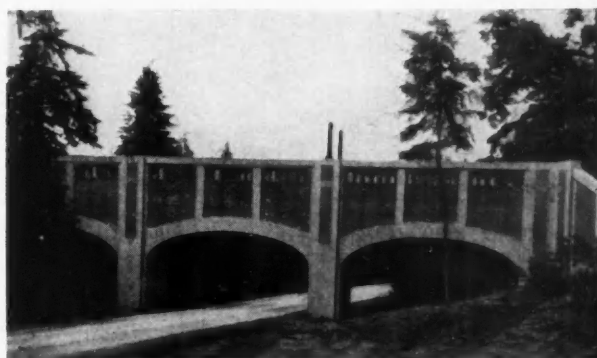
Artistic Viaduct Carries a 66-Inch Sewer Pipe
