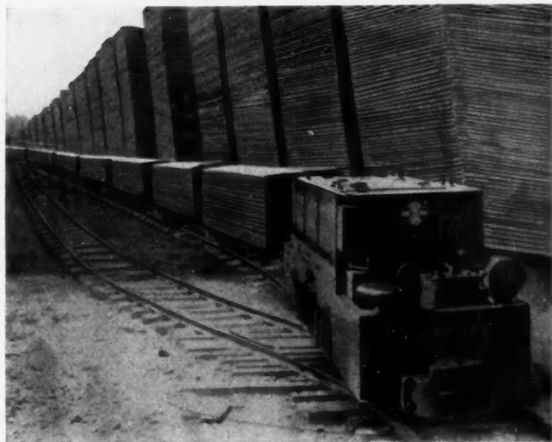
Electric Storage Battery Locomotive at Work in Big Lumber Yard
