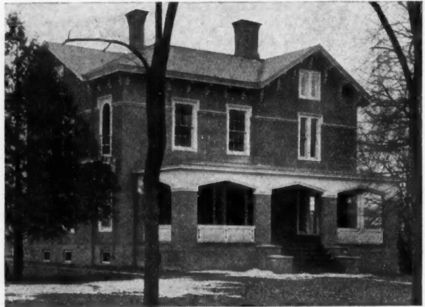
Fine House at Orange, N. J., Roofed as to Porch Roof and Deck with Con-Ser-Tex Canvas Roofing.
