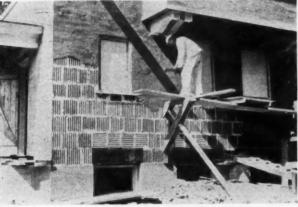
tile from the bottom of the After the tile walls were laid a cement plaster finishing coat basement up to the roof. was put on. This will never crack.
