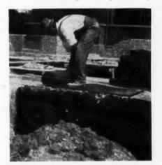
On top of the concrete foundation the men laid a damp proofing course of asphalt soaked paper to keep moisture from creeping up.
