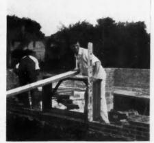
The masons had to do a lot of levelling and plumbing to get the window and door frames set just right.
