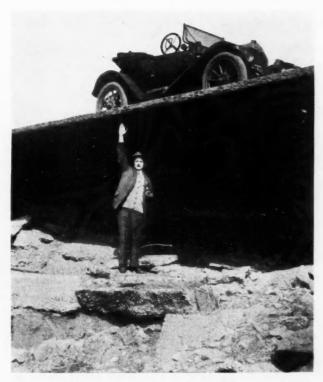
Despite the Fact That the Pavement Was Undermined to the Depth of Six and One-Half Feet, It Was Able to Bear Up Weight of an Automobile.
