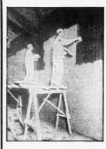
Hy-Rib steel sheathing combines in itself reinforcement, forms, lath and studs. Eliminates forms in concrete roofs and sidings, eliminates channels in partitions, ceilings, furring, etc. Also used in culverts, tanks, silos, etc.
