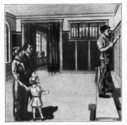
Utility can be laid satisfactorily—even in the coldest weather by nailing direct to the studding or on top of old plaster.
