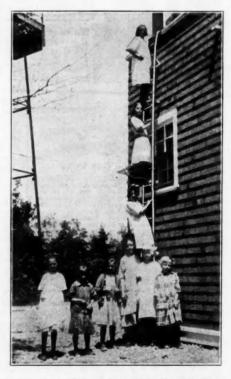
The "Kingsteel" Fire Ladder is Built with Heavy Steel Forgoings and is Treated so that it is Rust Proof.
