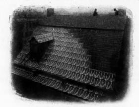
Old Wooden Roof Covered Over with National Sheet Metal Shingles.
