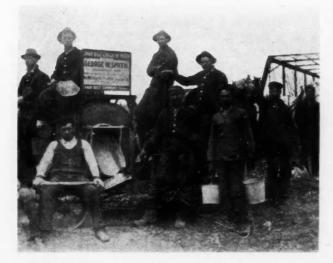
Bridge Work is Profitable When Done with a Power Mixer. Contractor Geo. W. Smith, of Belleville, Ohio, and His Crew Discovered After Just Finishing a County Road Bridge with the Help of a "Chain Belt" Mixer that Averaged 100 Cubic Yards of Mixed Concrete Per Day.
