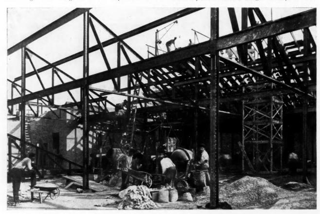
J. C. Davidson, Ex-Carpenter and Carpenter-Contractor of Columbus, Ohio, Successfully Handling Entire Construction on Extra High-Grade New Factory Building for the Columbus Die & Tool Company. He Has in Use Two "Big-an-Litle" Concrete Mixers on This Job, Mixing Both Concrete and Mortar, and Operating Material Hoist. This is a One-Story, Saw-Tooth Roof Shop Building; Has Sub-Floor of 8-inch Concrete and a 2½-inch Thick Concrete Roof.
