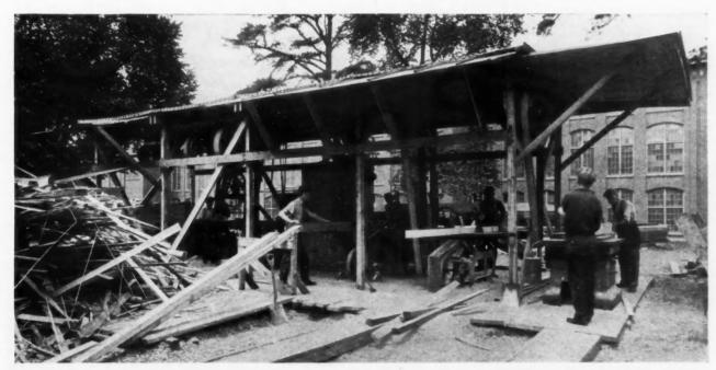
Close View of Carpenter Shop Equipped with Four Power Saws, Planer, Emery Wheel, and Wire Twister as Used for Making Concrete Forms for Cheney Bros. New Silk Mill, South Manchester, Conn.
