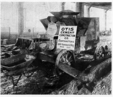
A Double Trough "Hartwick" Continuous Mixer Laying 150,000 Square Feet of Concrete Floor in the Detroit-Paige Motor Company's New Factory, Detroit, Mich. The Otis Cement Construction Company, Contractors. This Machine has been in Hard, Continuous Service for Seven Years.
